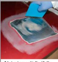
4 Apply and remove a thin film of ProWorx filler (Known as a wetting up coat), mix the removed product back into your existing filler.
