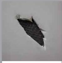
**3** Cut a piece of Aluminium mesh to the approximate size of repair. Secure the mesh in place ready for the filler application.
