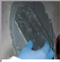
8 Apply the Plex to the fabric webbing and then apply with a firm even pressure to the reverse of the repair area.
