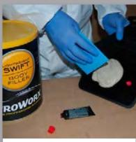
**7** Once the area has been prepared mix your ProWorx filler with hardener at a ratio of 2% at an ambient temp of 20°C.
